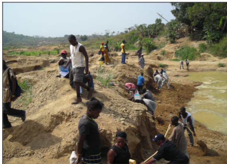
Re-routing a stream bed in Tankoro, Kono District
